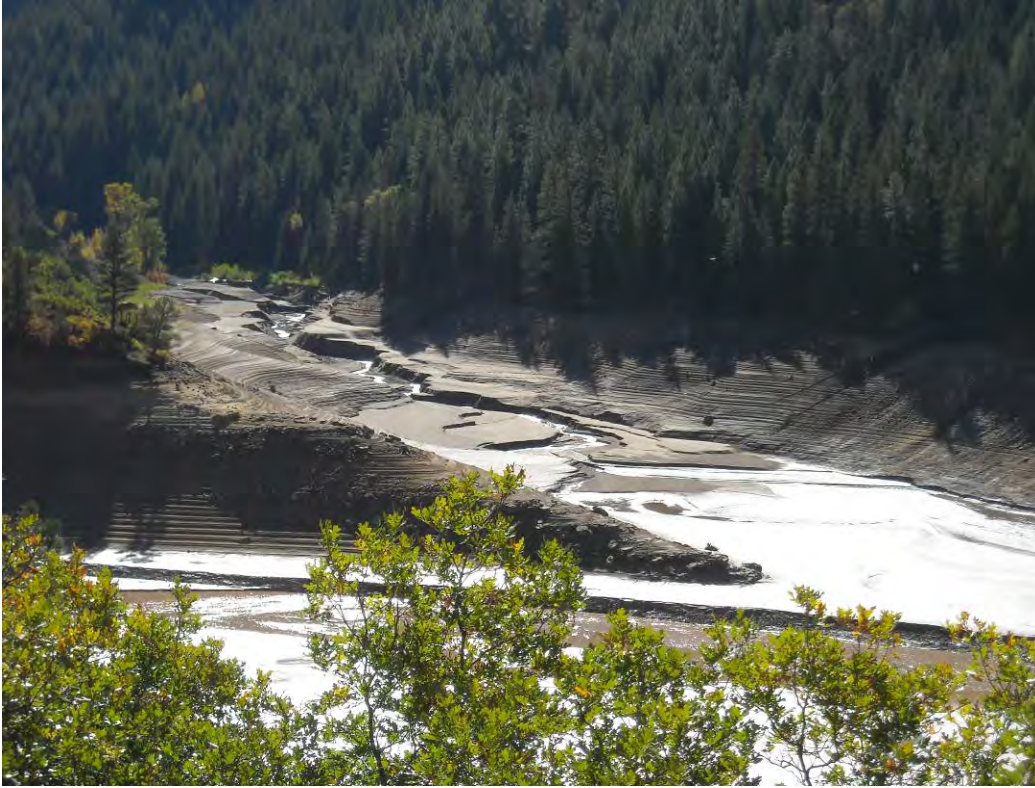
Figure 9-63. A photo of Paonia Reservoir in Colorado after the reservoir is drawn down showing how a channel incised through a portion of the reservoir sediments .
