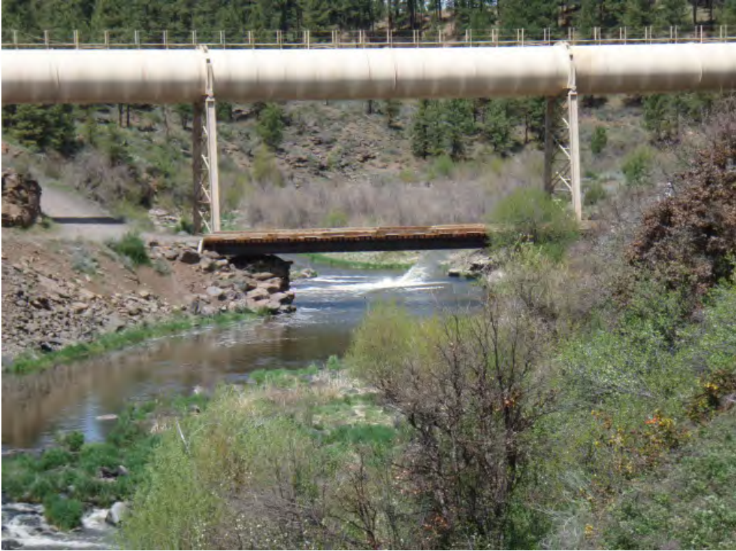
Figure 10-9. J.C. Boyle Bypass Reach Bridge.
