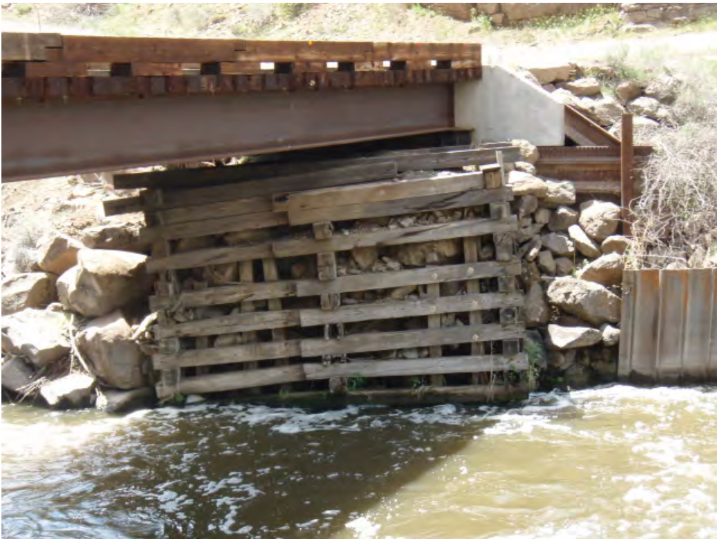
Figure 10-10. Abutment of J.C. Boyle Bypass Reach Bridge.
