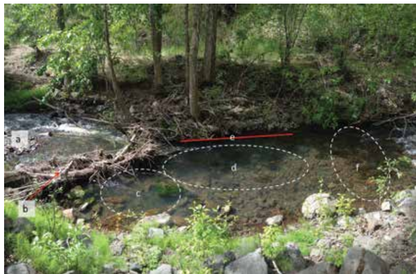
Figure 6. Example of changes to a plane-bed section of stream after construction of a large woody debris (LWD) structure: (a) bank-attached bar, (b) LWD structure, (c) eddy pool, (d) convergent hydraulic jet and scour pool, (e) new undercut bank, and (f) riffle bar.
